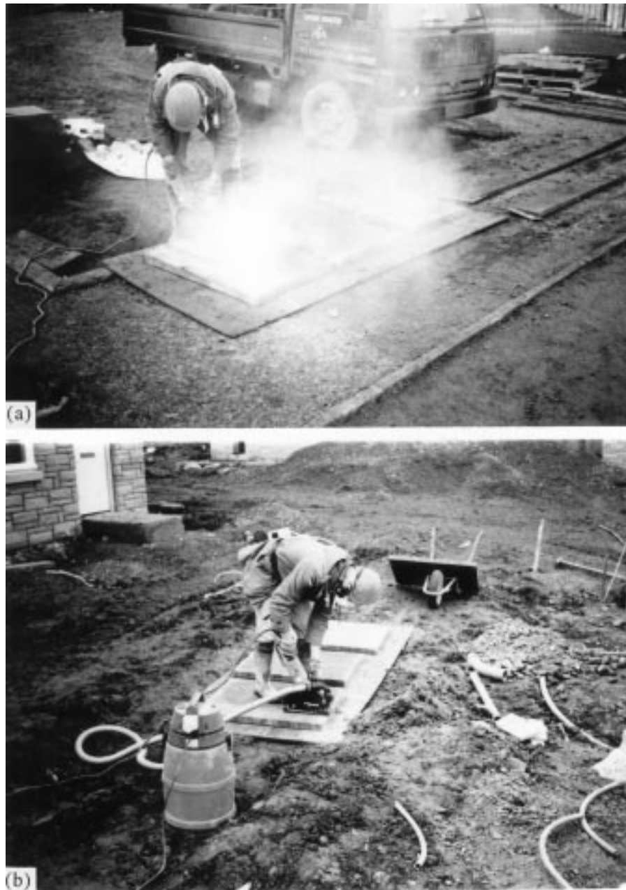
Fig. 2. Slab cutting with pressurised water tank system. (a) Without control; (b) with control.
