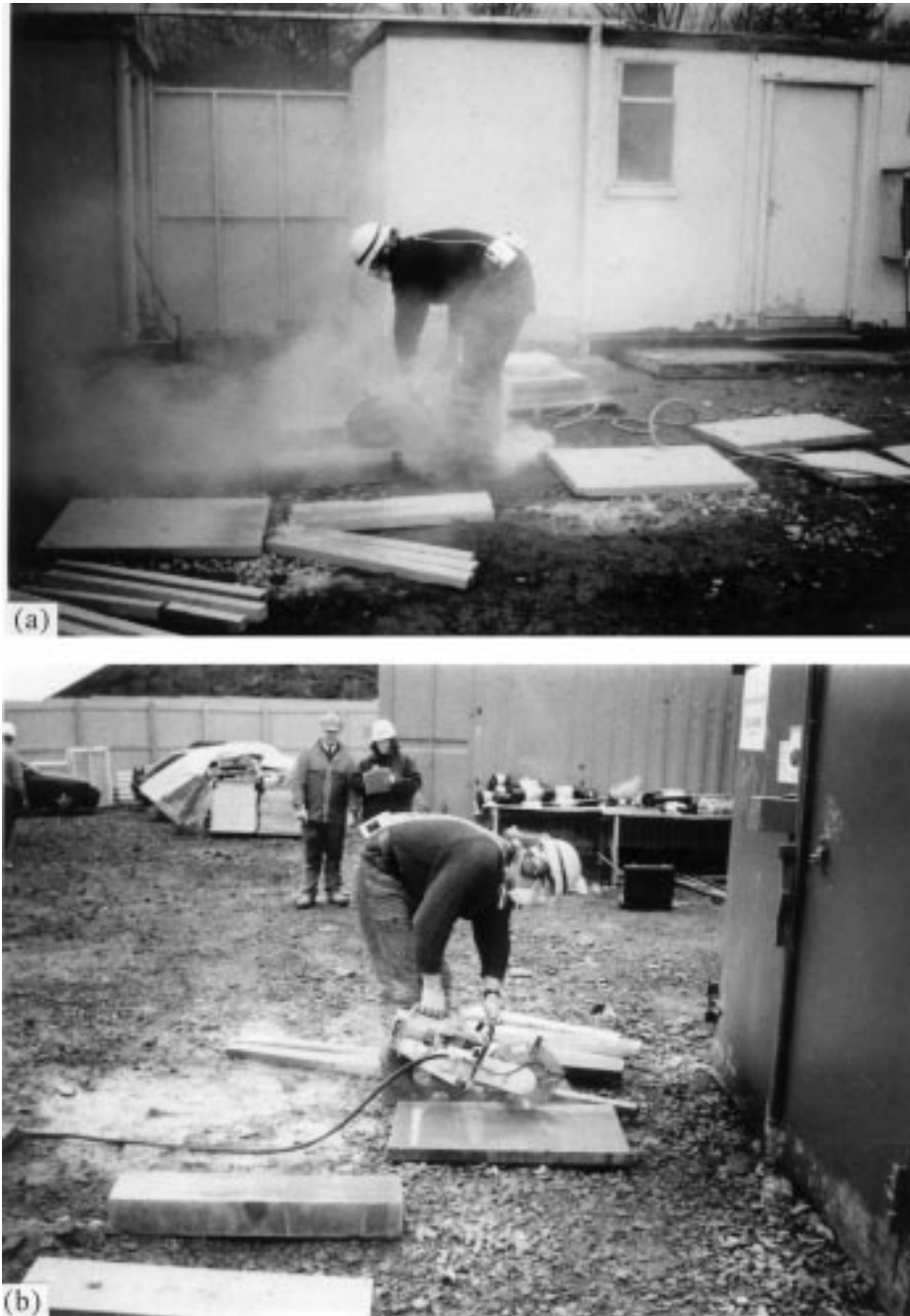
Fig. 3. Slab cutting with LEV system. (a) Without control; (b) with control.
